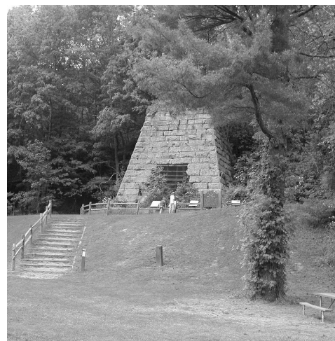
Hope Furnace at Lake Hope State Park
